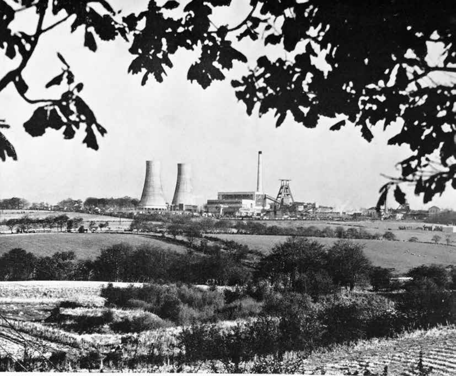
BARONY POWER STATION, AUCHINLECK
