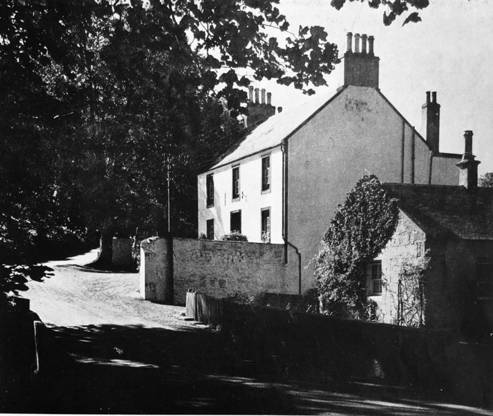
STAIR INN, COYLTON.
